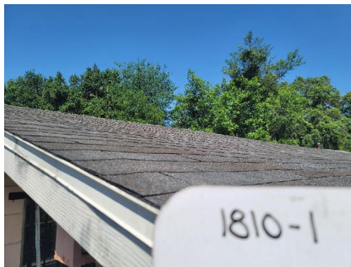
1810-1 Asphalt Shingle/Tar Typical Exterior Roof
